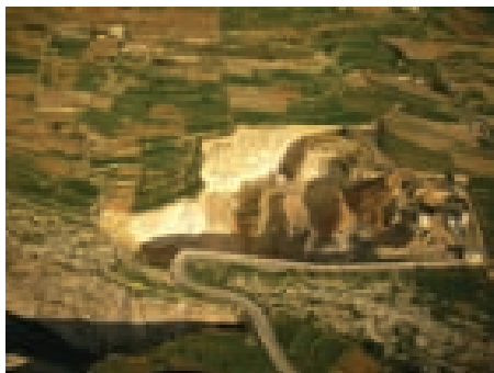
Figure 15. Active hardstone (Coralline limestone) quarry producing crushed gravel and sand for concrete slurries – Ghar Lapsi
