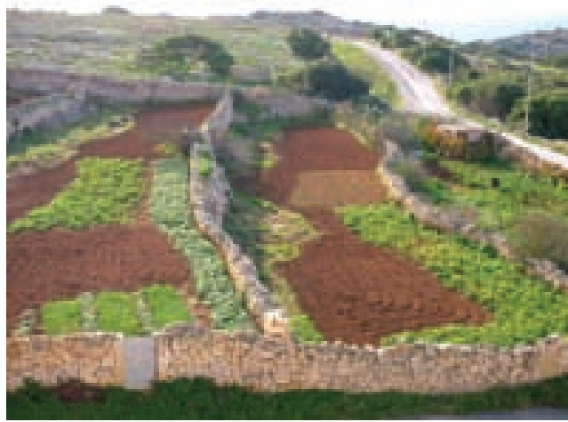
Figure 6. A typical example of a dry rubble wall armouring a terrace slope
